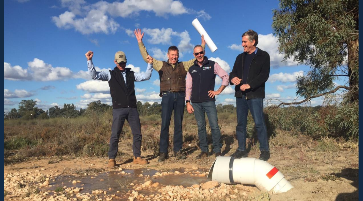
Celebrating the extended Renmark Irrigation Trust infrastructure being turned on to water Bookmark Creek floodplain, SA.
